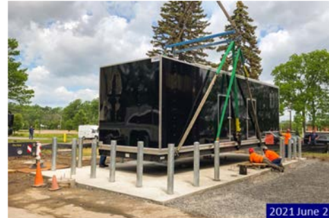
Generator and switchgear replacement
